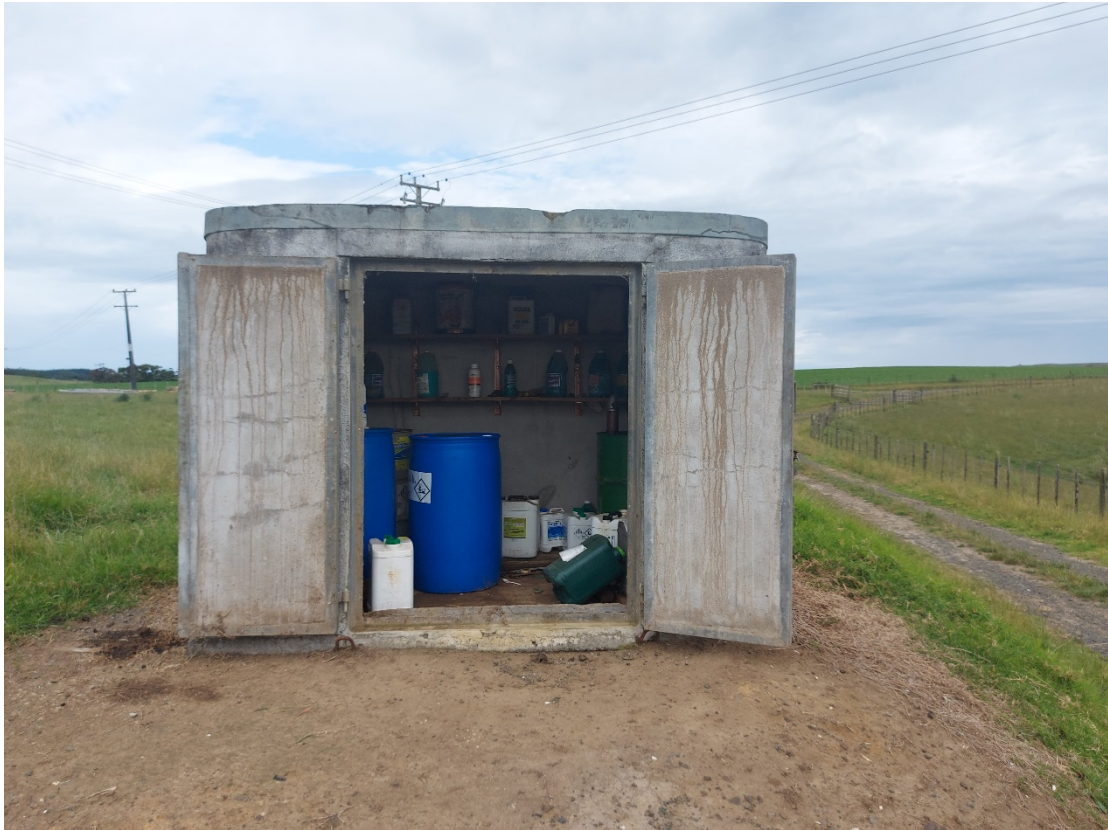
Photograph 5: Photograph showing the bunded concrete hazardous chemicals storage shed.
