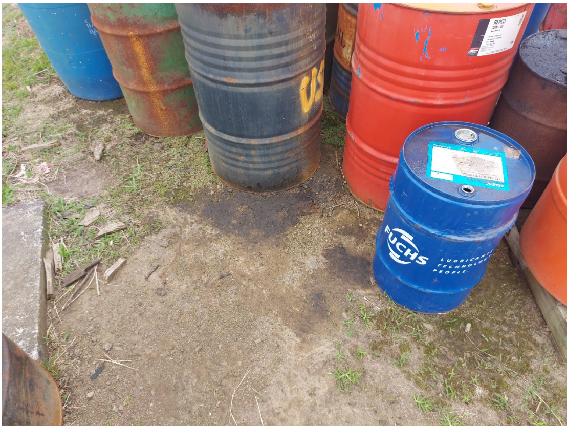
Photograph 8: Staining on ground surrounding un-bunded storage of fuel/oil drums next to ASTs.
