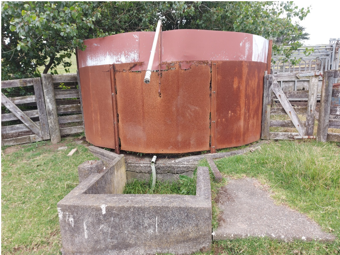
Photograph 10: Old shower sheep dip in yard area next to woolshed.
